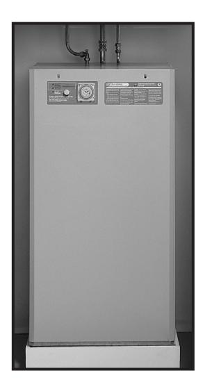
Your SysteMate 2000 is a highly advanced Thermal Storage System which incorporates the latest in microprocessor technology to monitior your system automatically and ensure it operates at maximum efficiency. This includes periodically 'spinning' the heating pump to prevent seizing during prolonged unused heating periods.
